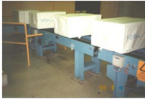
Straight conveying line for single bales.
